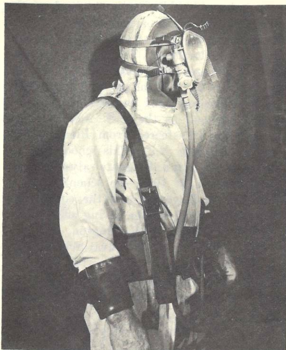
FIGURE 1-8.—Surface-supplied apparatus: lightweight diving outfit.
